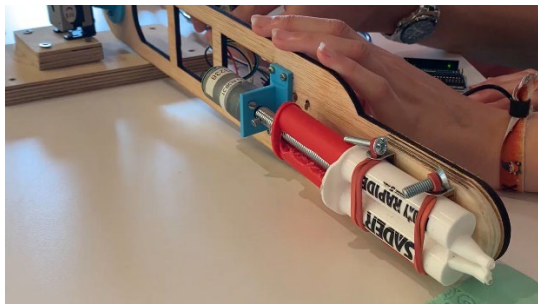
Figure 9. Development of a system to repair leaks areas in gas pipes
